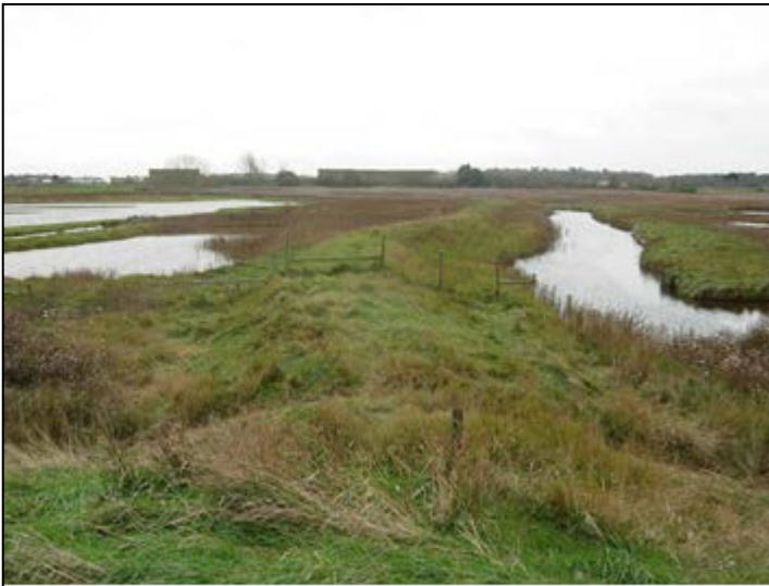
Raised bank at Delacroix - photo taken 14 November 2015
